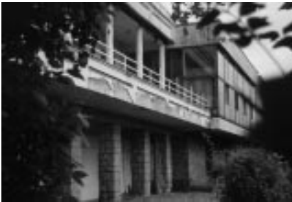
2.1. Kahlenberg restaurant in Vienna - Döbling, architect: Erich Boltenstein, 1935. Photo: B. Maldoner.
