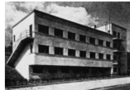
3.3. Settlement, Young Persons Home in Vienna - Döbling, architect: Anton Brenner, 1930. Contemporary photo.
