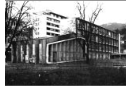
1.3. Old Textile School in Vorarlberg – Dornbirn, architects: Willi Ramersdorfer - German Meusburger, 1958. Photo: Bundesdenkmalamt.
